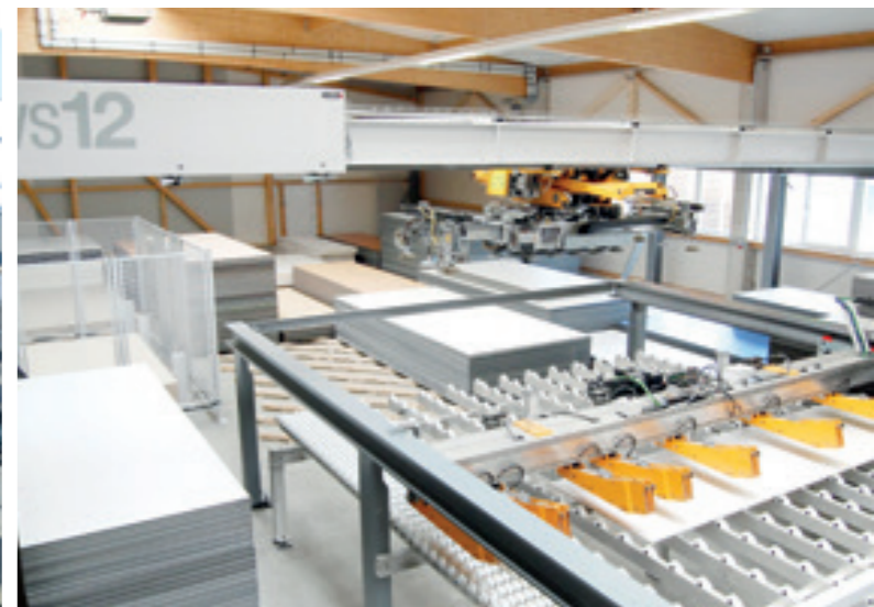
Area storage system: Increased productivity
